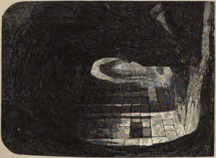
Tunnel along Western Basement Wall (Nimroud)
