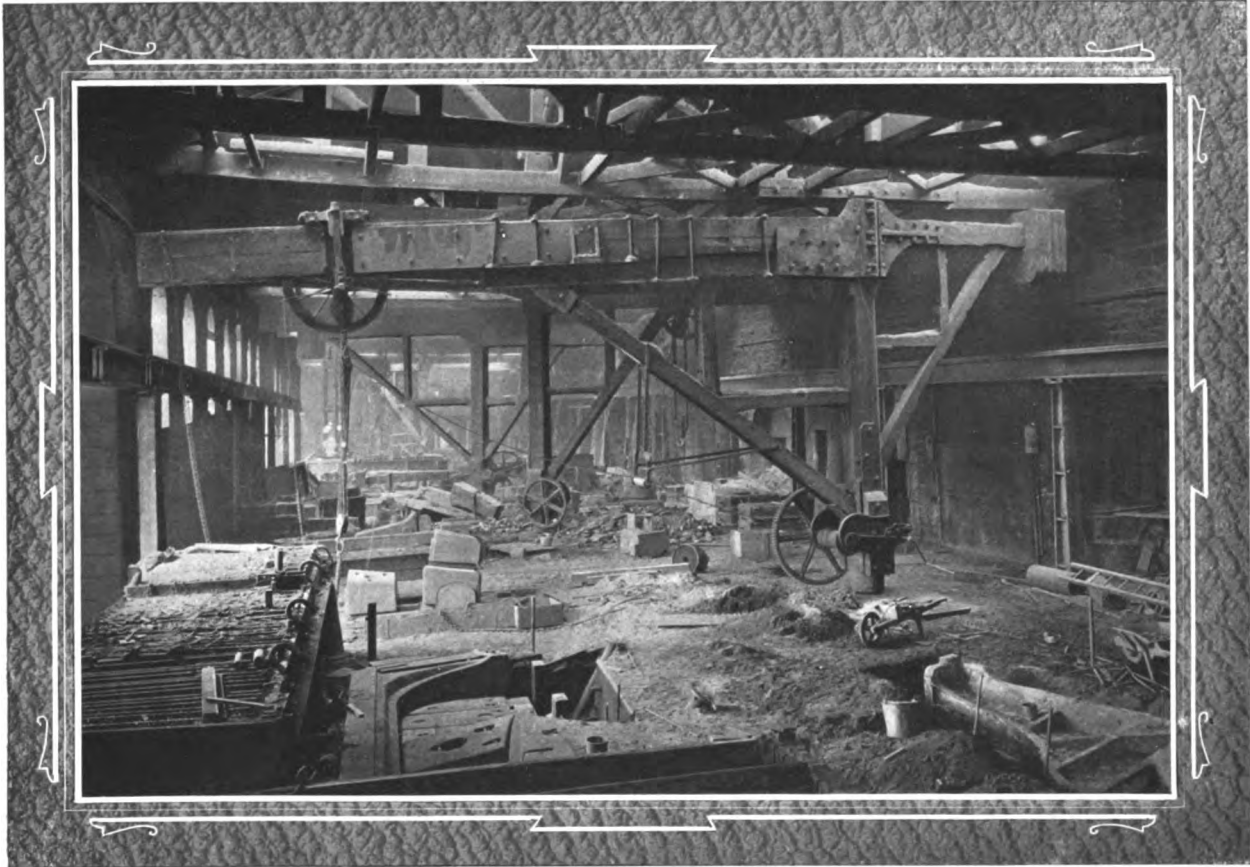
OLD FOUNDRY, LOWMOOR IRON WORKS.
